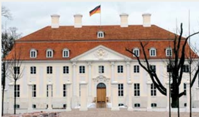
▲ The restoration of historic buildings requires top-notch engineering and technical solutions that preserve the unique character.
